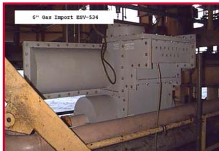
The cast epoxy systems are manufactured using a moulding technique base on information taken from CAD models or site survey. The pre-formed components are then simply bolted in place on the risers, valves or actuators, sealing all joints against water ingress
